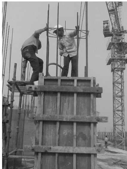
Fig. 11.2: Form work for column
