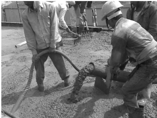
Fig. 10.4: Pouring of RMC
