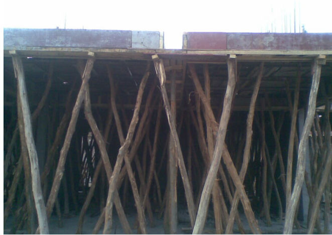
Fig. 11.3: Ballies below wood planks
